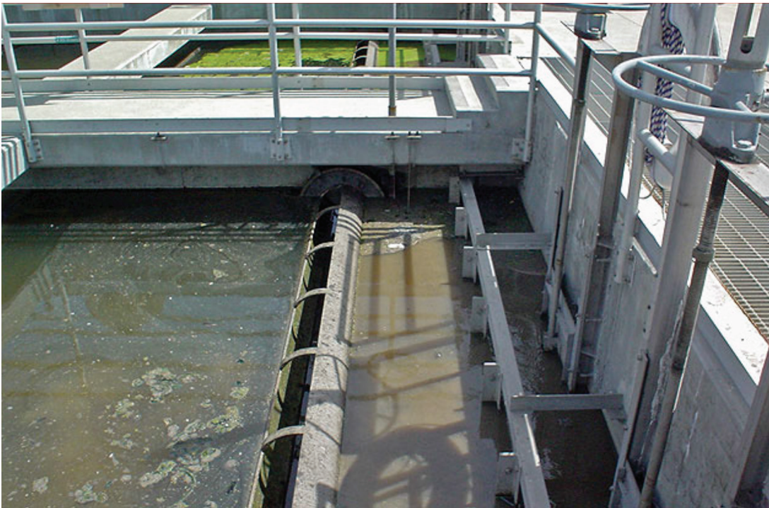
FIGURE 12.3 Rotating scum trough (courtesy of Jim Myers & Sons, Inc., Charlotte, North Carolina).
