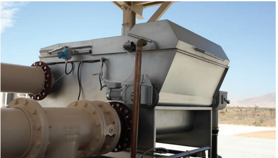
FIGURE 12.6 A photograph of a M2R microscreen for raw wastewater treatment (courtesy of M2 Renewables, Lake Forest, California).
