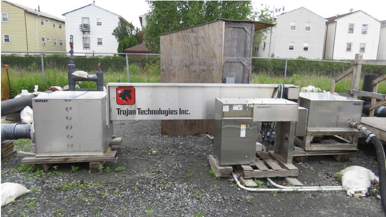
**Figure 2. Trojan UV3000 unit on project site**
